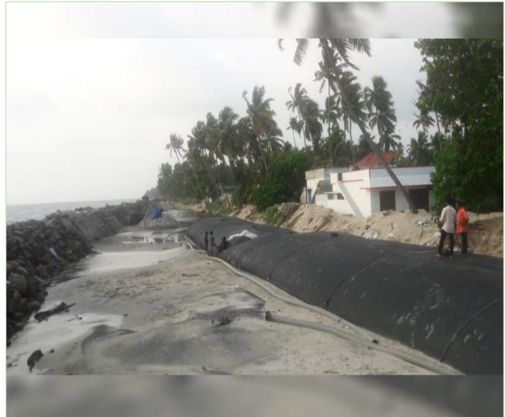
GEOTUBE PROJECT IMPLEMENTED WITHOUT SCIENTIFIC STUDY IN INDIA
