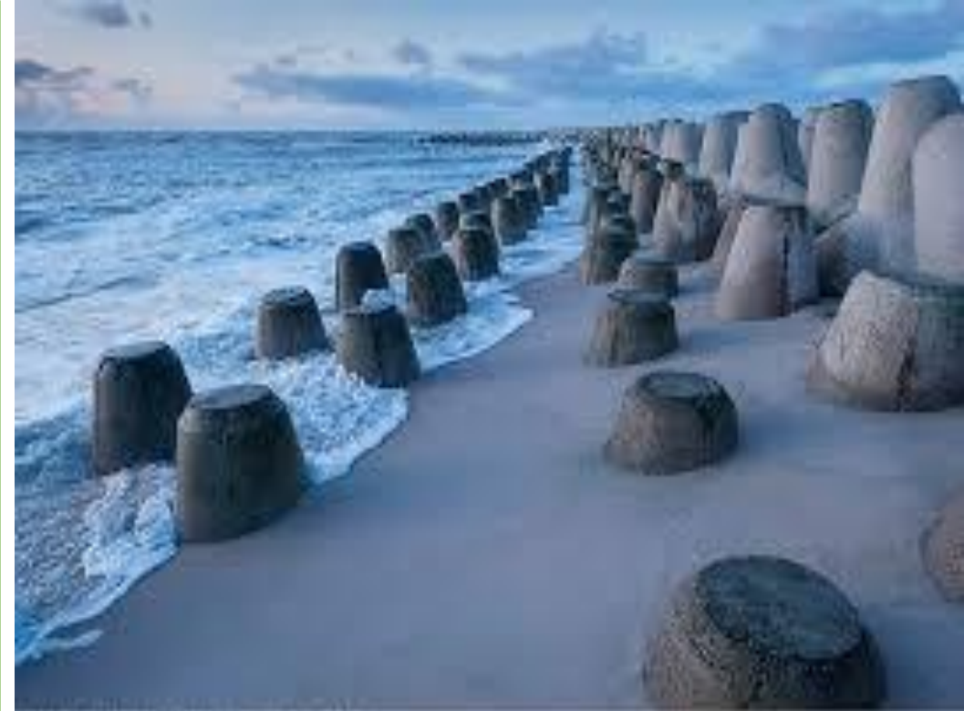
TETRAPOD SINKING IN BEACH SAND
